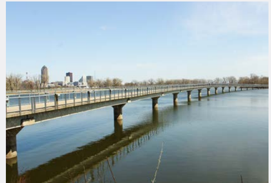
Gray's Lake Bridge, Des Moines, Iowa
