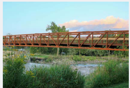
Mill Pond Pedestrian Bridge, Nora Springs, Iowa
