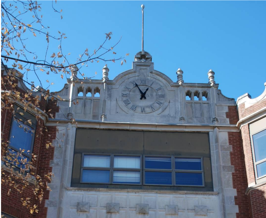
Photograph: 215 3rd St NW, entrance bay details, looking west, Marlys Svendsen, photographer, 11/16/2011.
