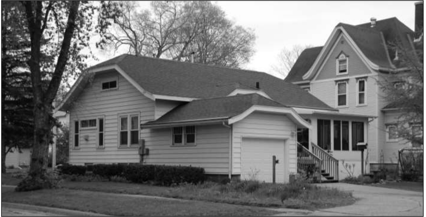
Sewell Rental House photo, 302 2 nd St SW, looking southeast (Svendsen Tyler, photographer, 2015)
