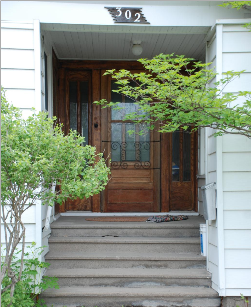
Photograph: 302 2 nd Street SW, entrance detail looking west, 4/7/2014, Andrew Bell, Svendsen Tyler, photographer.
