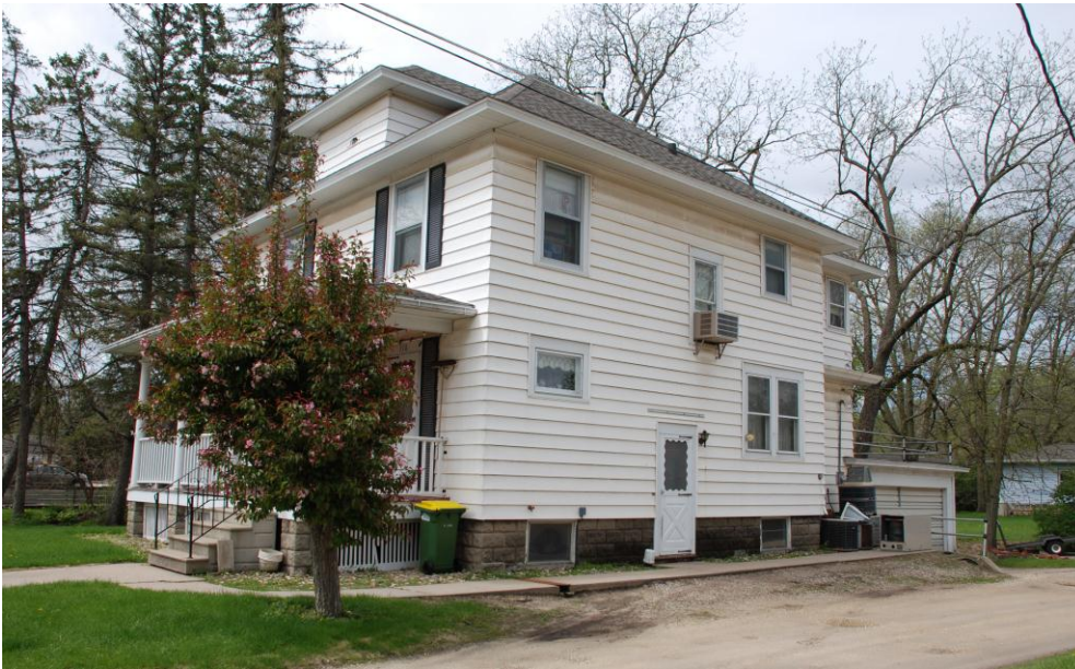
Photographs: 318 3 rd St SW, looking southwest and garage, looking southwest at rear of house, 5/15/2014, Marlys Svendsen, Svendsen Tyler, photographer.
