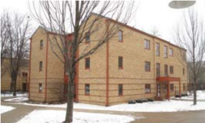
South Hall looking northeast
