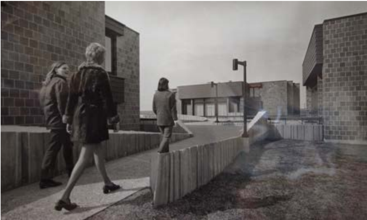
Figure 46. Waverly Manor (Map #9-13) built in 1969 on the north edge of campus to west of Afton Manor (Wartburg College Archives Photograph Collection)
