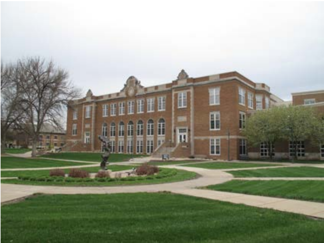
Photograph 16. Luther Hall (#21), camera facing northeast
