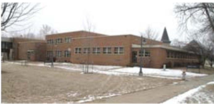
Fine Arts Center, looking northeast
