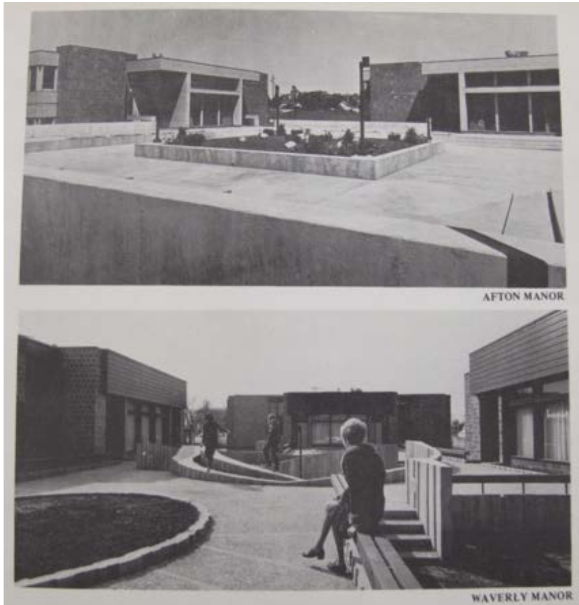
Figure 45. Courtyards in two dormitory clusters, Afton Manor (Map #4-7) and Waverly Manor (Map #8-11), built north of 5 th Ave NW on the north edge of campus (Ottersberg 1977: 24c)
