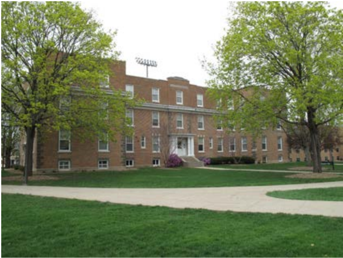
Photograph 3. Grossman Hall (now Founders Hall) (#2), camera facing northwest
