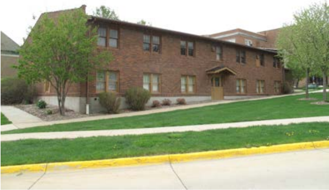
Photograph 19. Little Theater (original gymnasium), camera facing northwest
