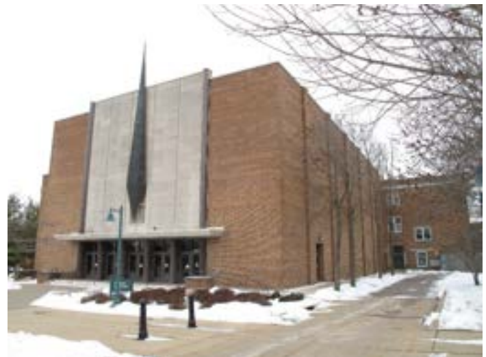
Neumann Auditorium addition, looking southwest
