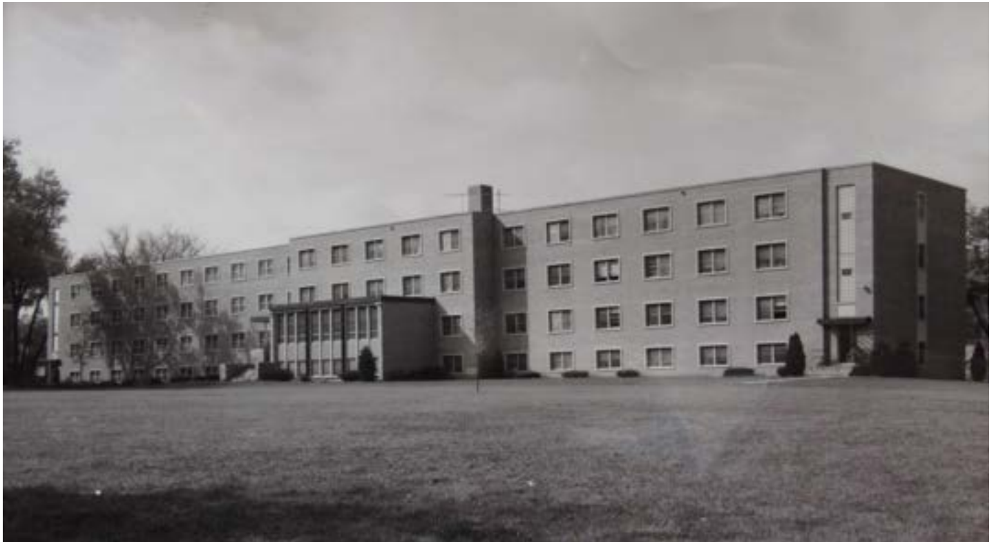
Figure 39. Addition to Clinton Hall (at left) and original building (at right), looking southwest (Wartburg College Archives Photograph Collection)
