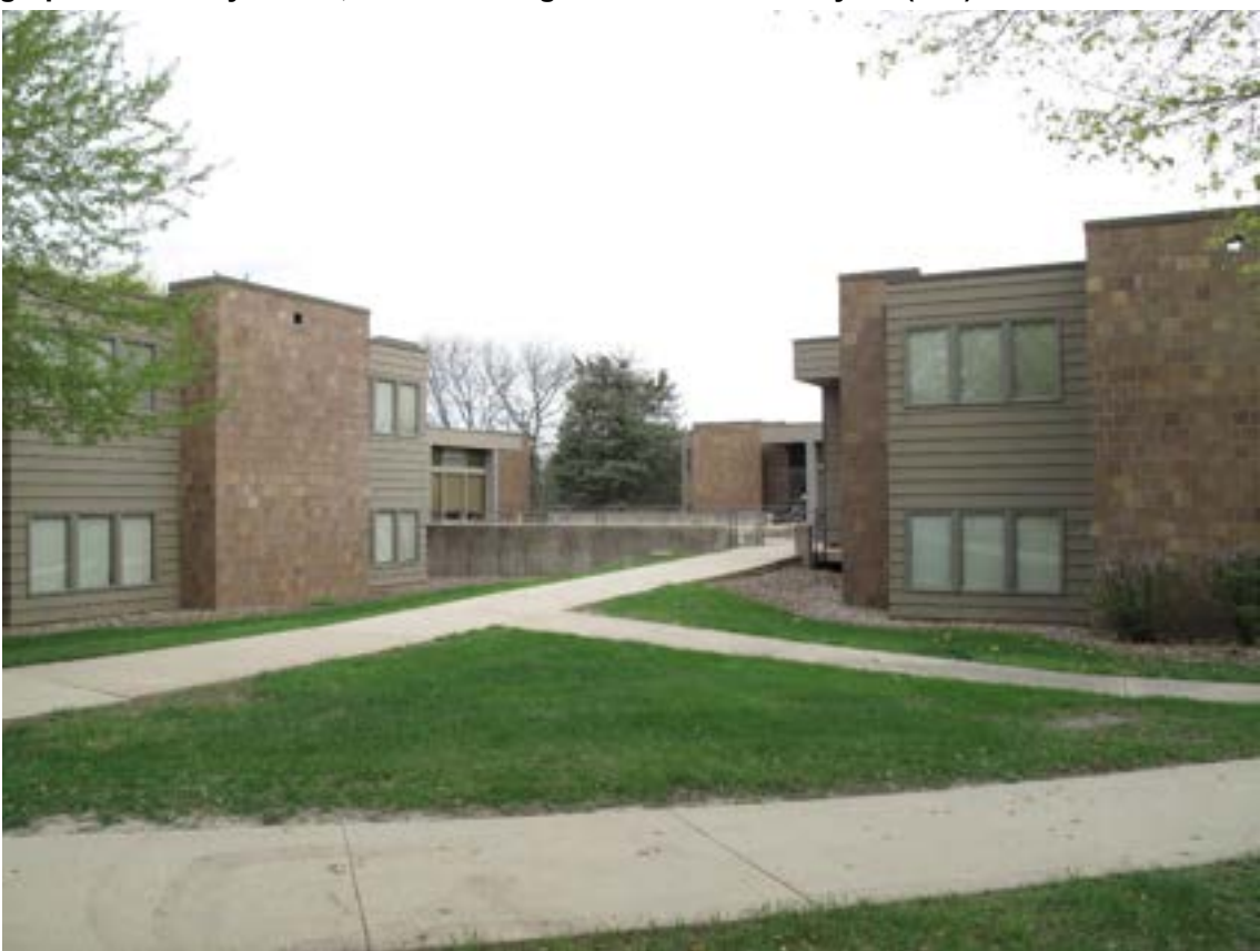
Photograph 8. Afton Manor (#4-8), camera facing northwest
