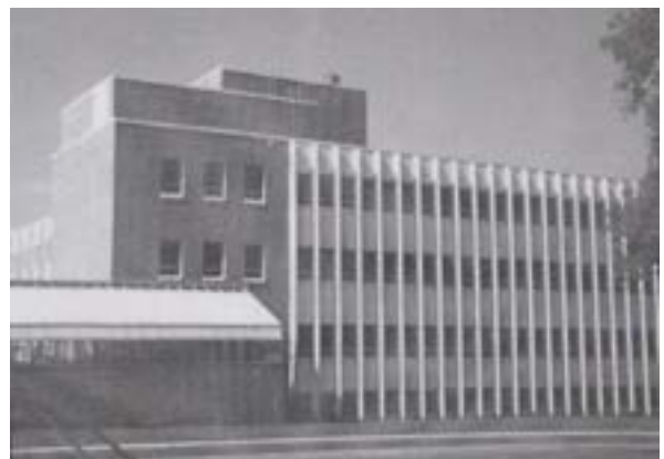
Becker Hall of Science in June 1968, looking northeast (Waverly Historical Photograph Collection)
