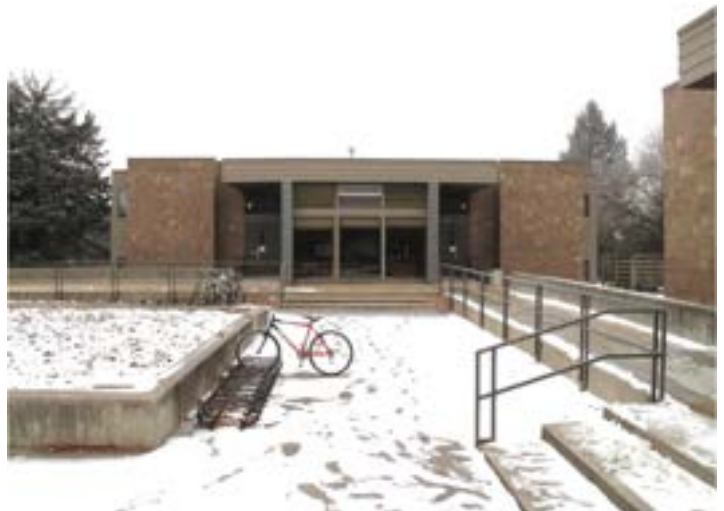
Ernst House, looking north
