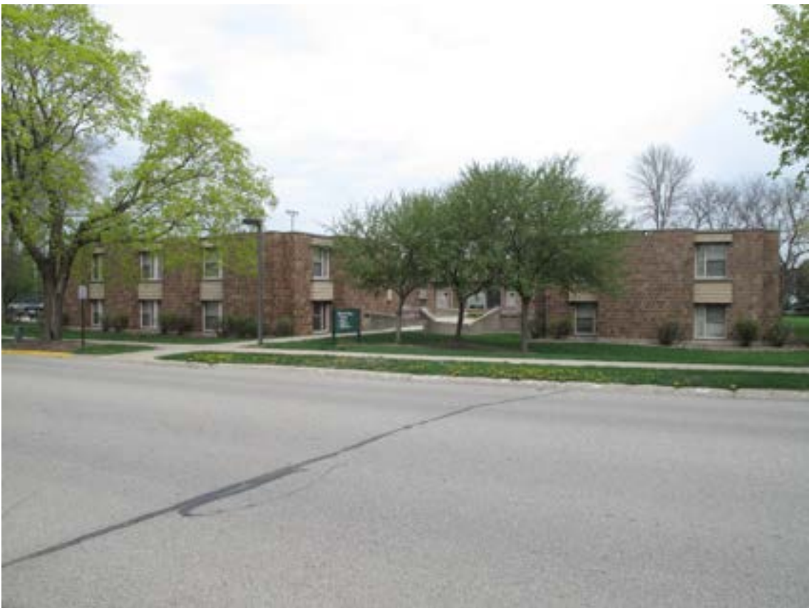
Photograph 6. Waverly Manor (#9-13), camera facing northwest
