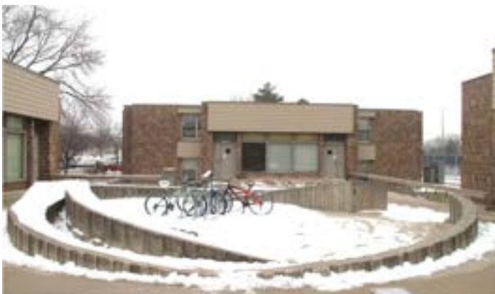
Otterburg House, looking southwest
