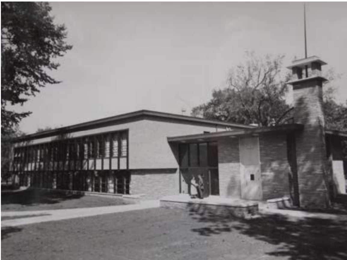
Figure 27. Student Memorial Union (core of Map #16) and Danforth Chapel (demolished), built in 1954-55 (Wartburg College Archives Photograph Collection)
