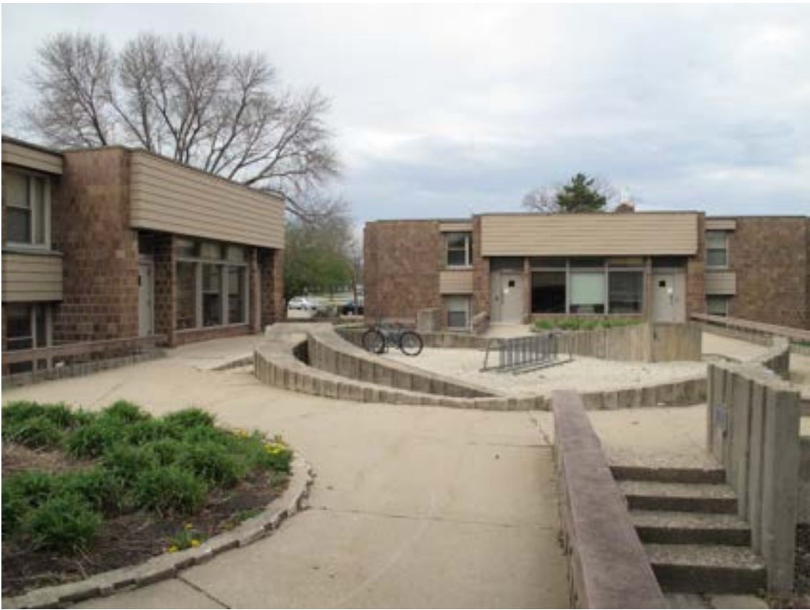
Photograph 7. Waverly Manor, camera facing west towards courtyard (#13) and Swensen House (#11)
