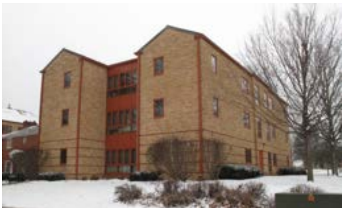
North Hall, looking southwest
