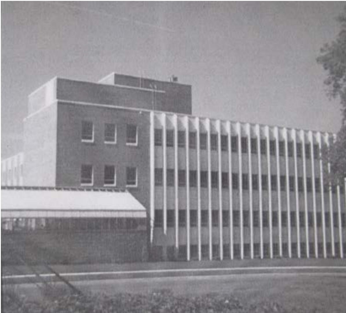
Figure 41. Becker Hall of Science (Map #22) in June 1968, looking northeast (Waverly Historical Photograph Collection)
