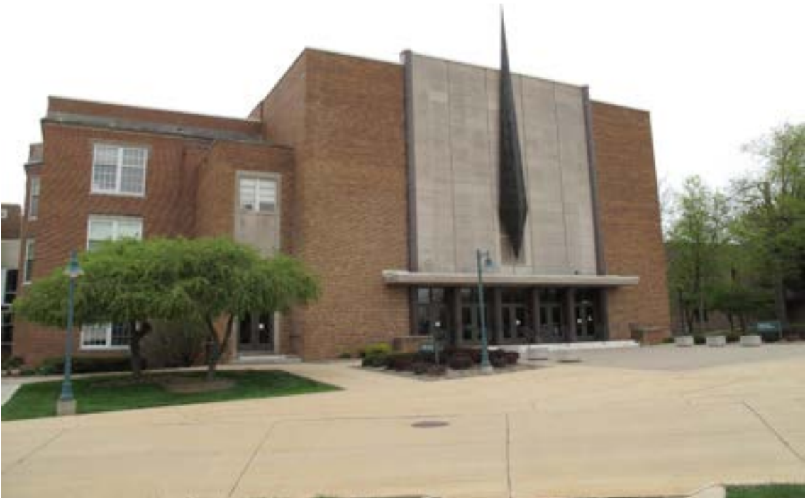
Photograph 18. Neumann Auditorium (rear of Luther Hall) (#21), camera facing northwest
