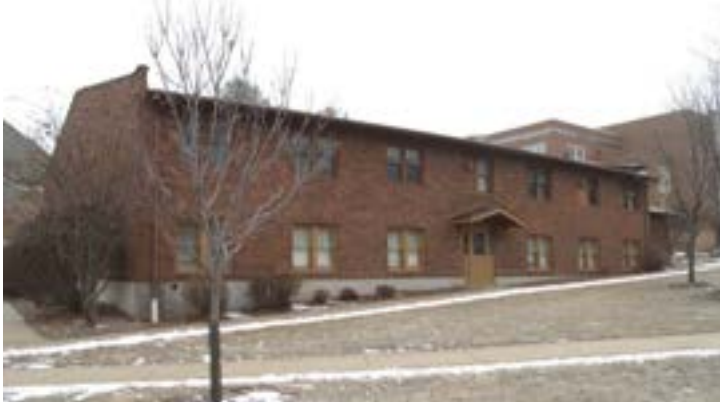
Little Theater, looking northwest
