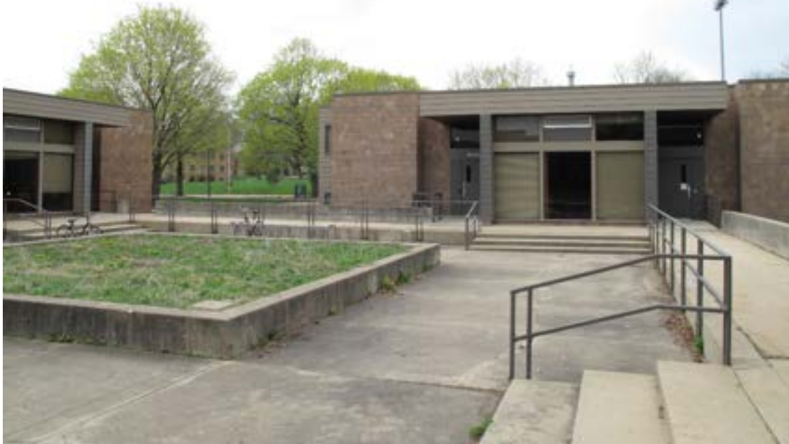
Photograph 9. Afton Manor, camera facing southeast towards courtyard (#8) and Cornils House (#7)
