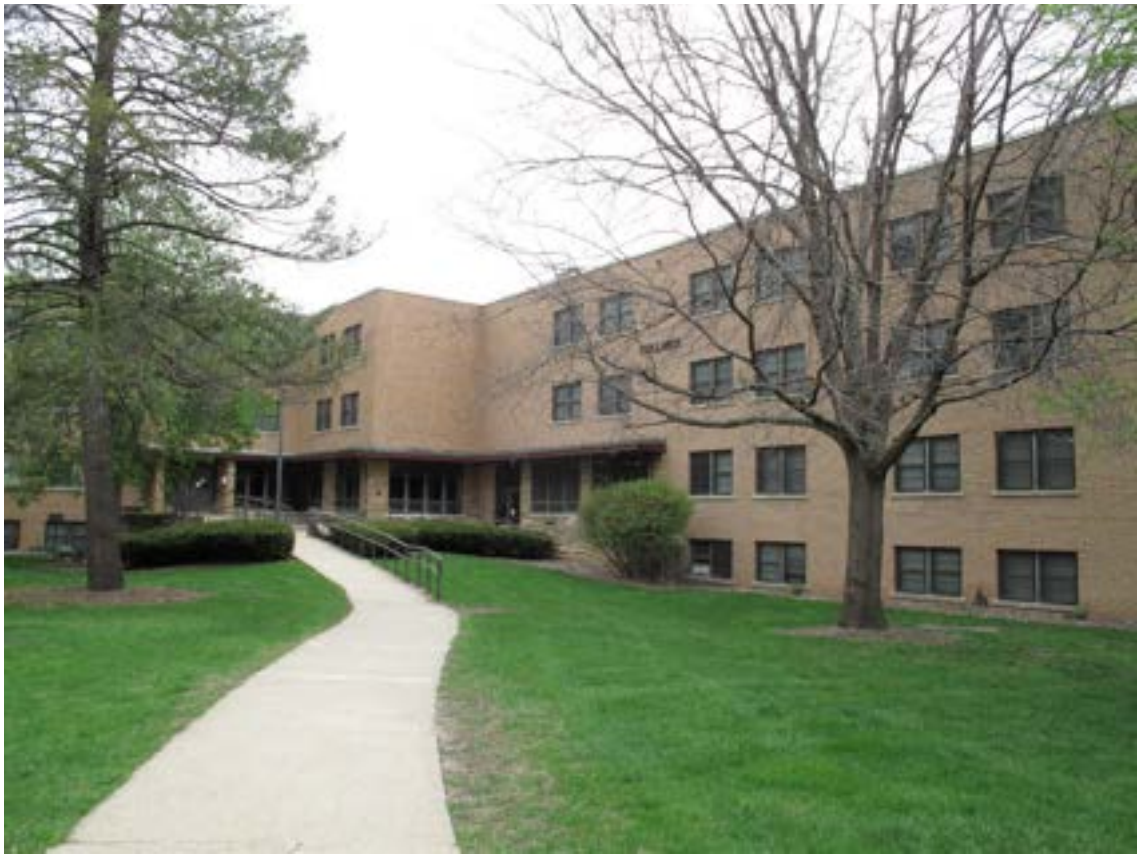
Photograph 11. Centennial Complex (#14), camera facing northeast to entry to Centennial Hall and Vollmer Hall
