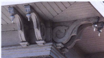
Decorative double brackets under the eaves
