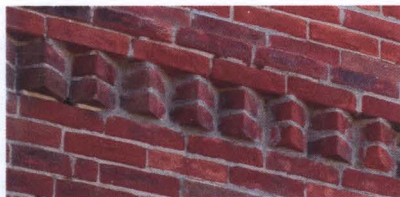
Course of sawtooth bricks
