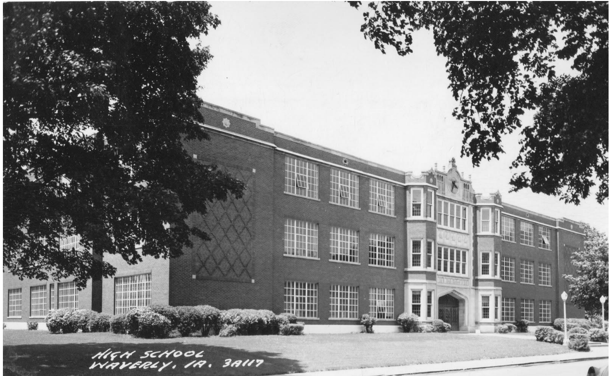
Photo showing the original windows.
