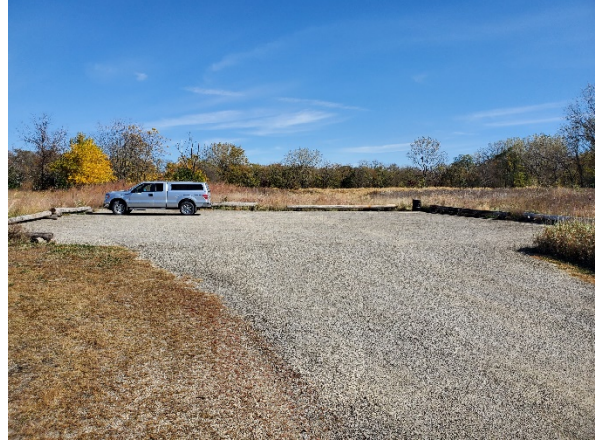
(Seal coated parking lot at Red Cedar)
