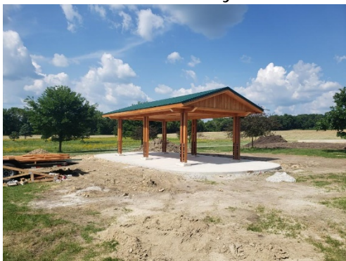
(Prairie Park Shelter almost complete)
