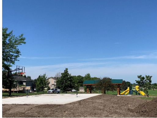
(Completed Prairie Park Project)
