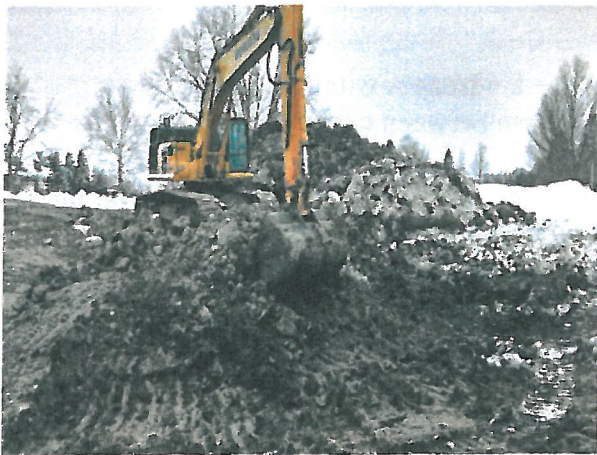
Removing muck from pond 4
