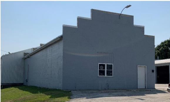
(View from the Rail Trail)
