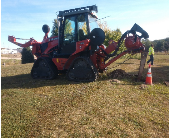
Pulled new irrigation wires for #3
