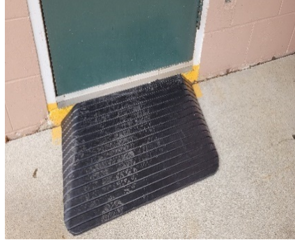
Eliminating a trip hazard by installing a mat at the Proshop.
