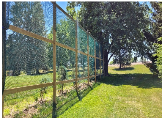
Installed safety fence between 9 & 5 tees.
