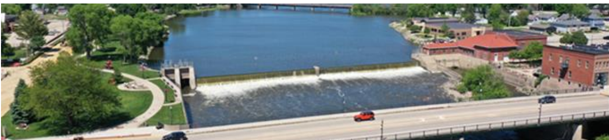
Aerial photo of the dam
