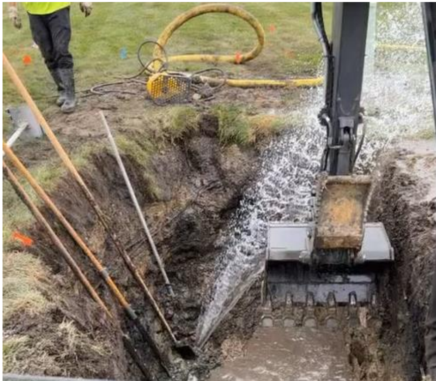
Water Division responds to a water main leak.
