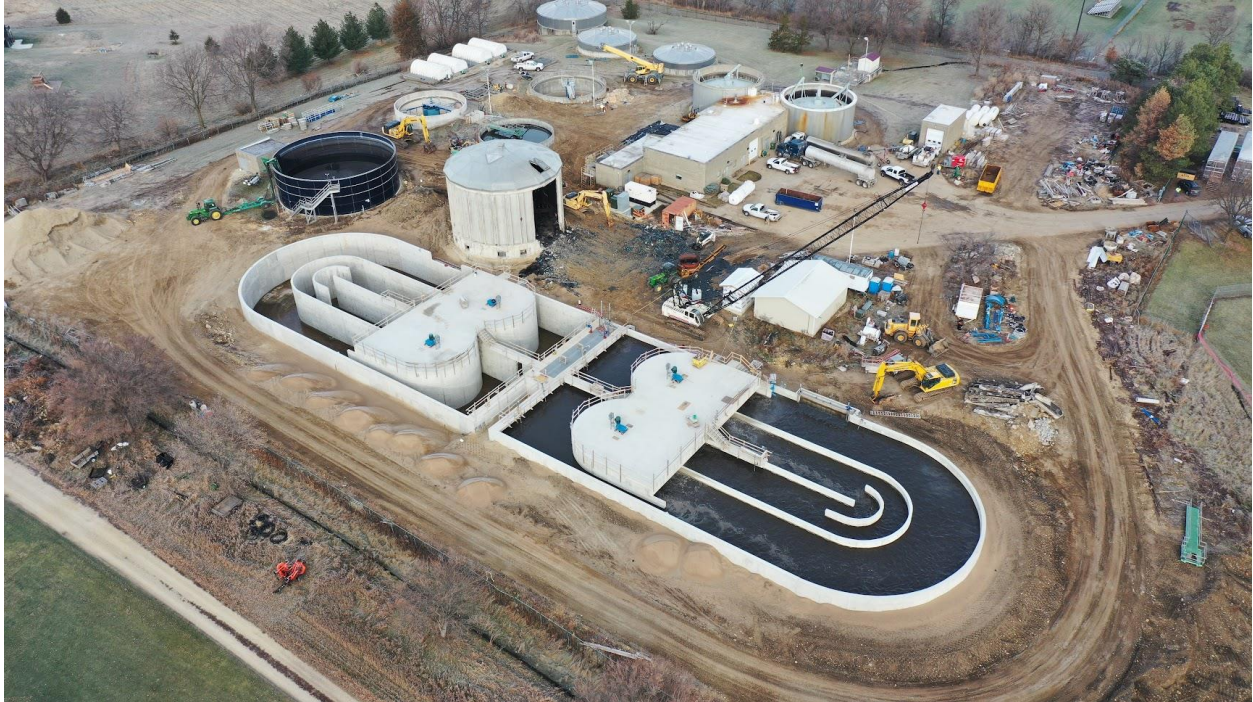
Aerial photo of the WPC Facility project in progress.
