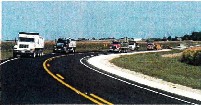
New: Final Pavement.
