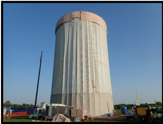
This is an example of the tarp system that will be used during the project.
