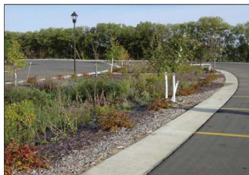
Example of using green infrastructure within a parking lot to capture run off
