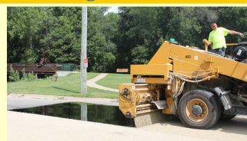
Contractor placing rock over oiled street. As soon as the rock has been placed on street, vehicles may drive slowly on the new surface.
