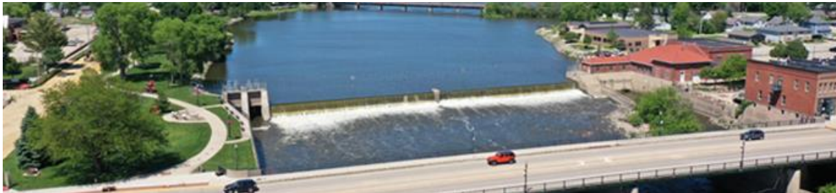
Aerial photo of the dam.
