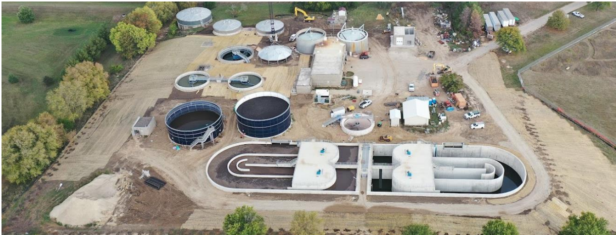
Aerial photo of the new WPC Facility.
