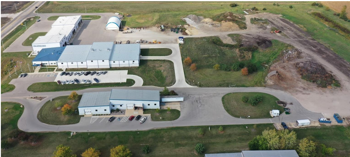
Pictured above: The Public Services facility is home to Public Works Administration, Streets, Solid Waste, Yard Waste Center, Recycling Center, Water, Sewer Line Maintenance, and Equipment Services.
