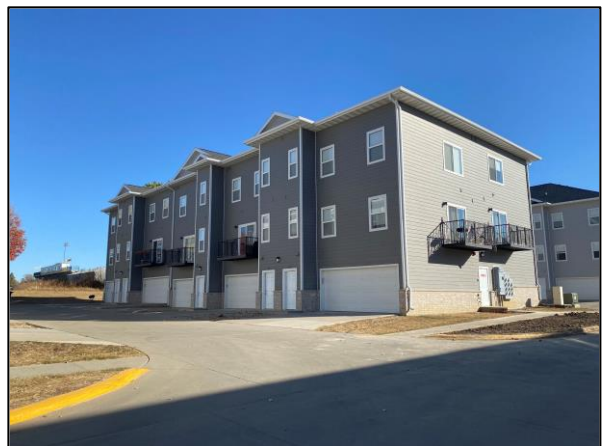
New construction multifamily rental
