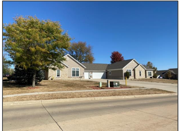
Attached single-family duplex units
