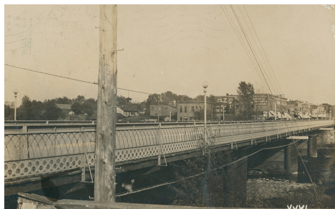
A view of the Bremer Avenue bridge. 1909
